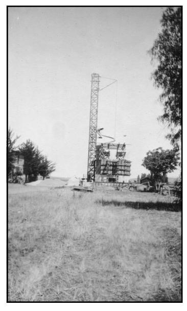
On August 1, 1918, the steel skeletal frame was being assembled before the pouring of the cement.
