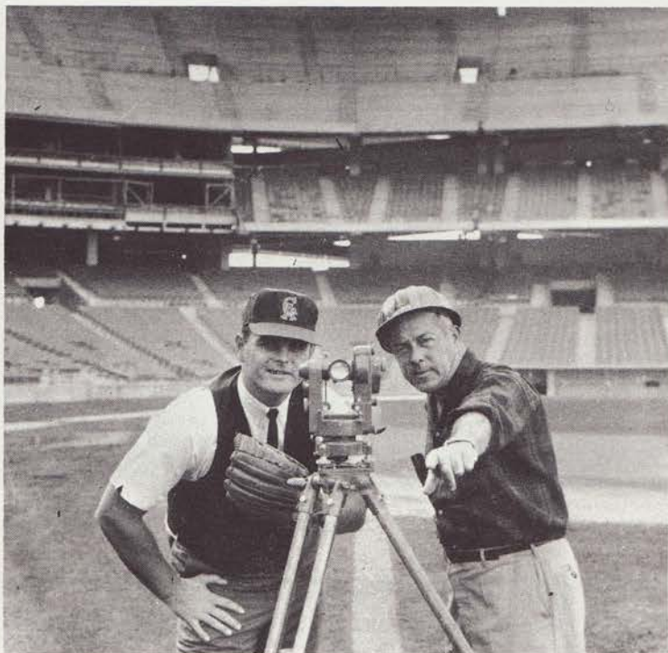
Drawing the line on home runs, Bob Lee sights down right field foul line, as California Angel relief fireballer gets briefing on future Anaheim Stadium home from Del E. Webb Corporation construction boss "Mac" McAllister.
