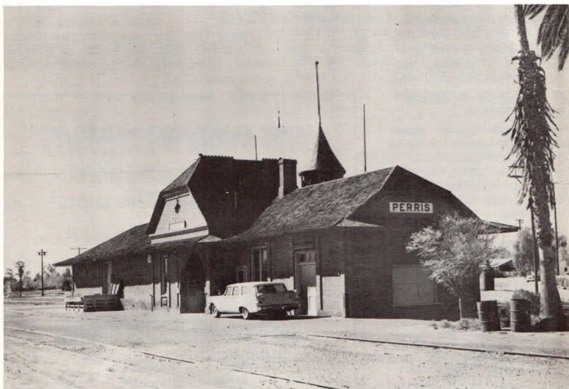
Front and rear view of Santa Fe's station in Perris which was erected in 1885. Badly in need of repair and a coat of paint Mayor Robert E. Warren has offered to make the railroad a swap, giving it permission to install a 50 by 160-foot stock pen at the south city limits in exchange for redecorating the depot.
