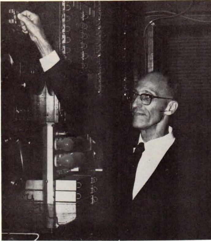
Not the "Hand that Rocks the Cradle" but the "Hand that Pulls the Switch". Knox Hager, telephone company executive, pulls switch at 11 p.m. Nov. 10, marking the end of the old Manual System and ushering in the new modern dial system.
